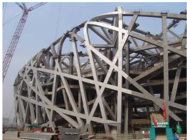
National Stadium under Construction
