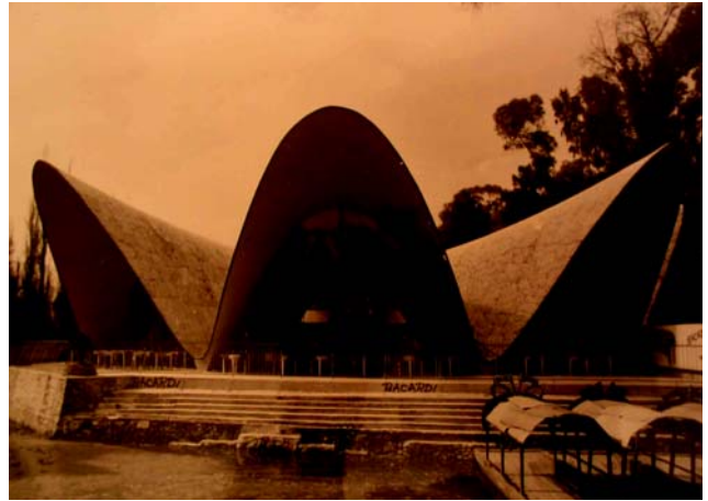
Figure 4.3. Photograph showing more diffuse shrinkage cracks after the structure has been completed
