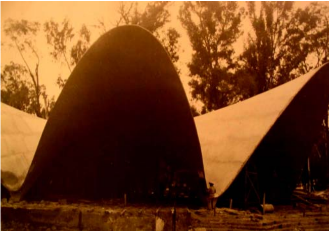
Figure 4.2. Photograph showing shrinkage cracks during construction. The cracks are most visible on the left side of the image.
